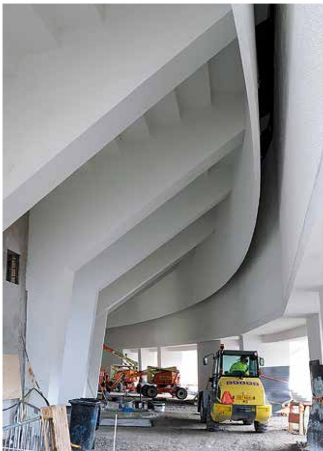
Fig. 10 The original 1938 circular wall inside the stadium building
