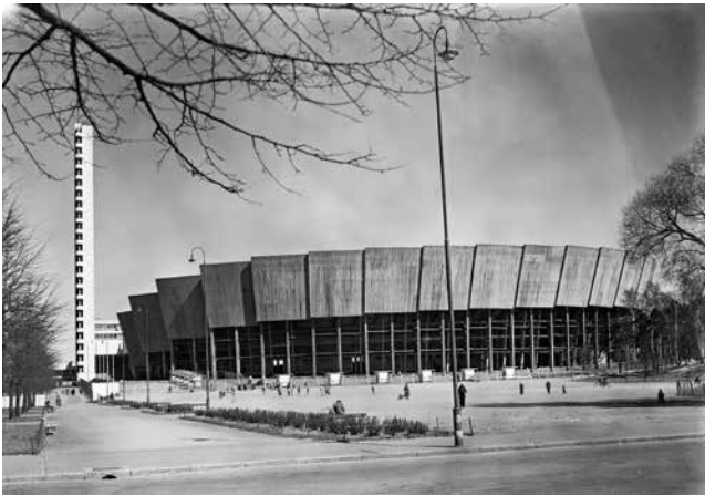
Fig. 3 The Helsinki Olympic Stadium in 1952
