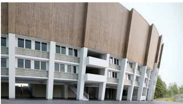
Fig. 6 The Olympic facade after its conversion, 2019; the new exit staircase 3rd bay
