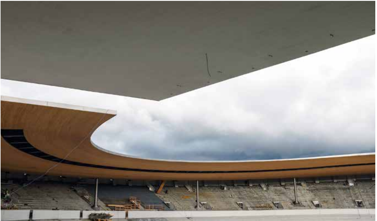
Fig. 5 The new canopy, 2019
