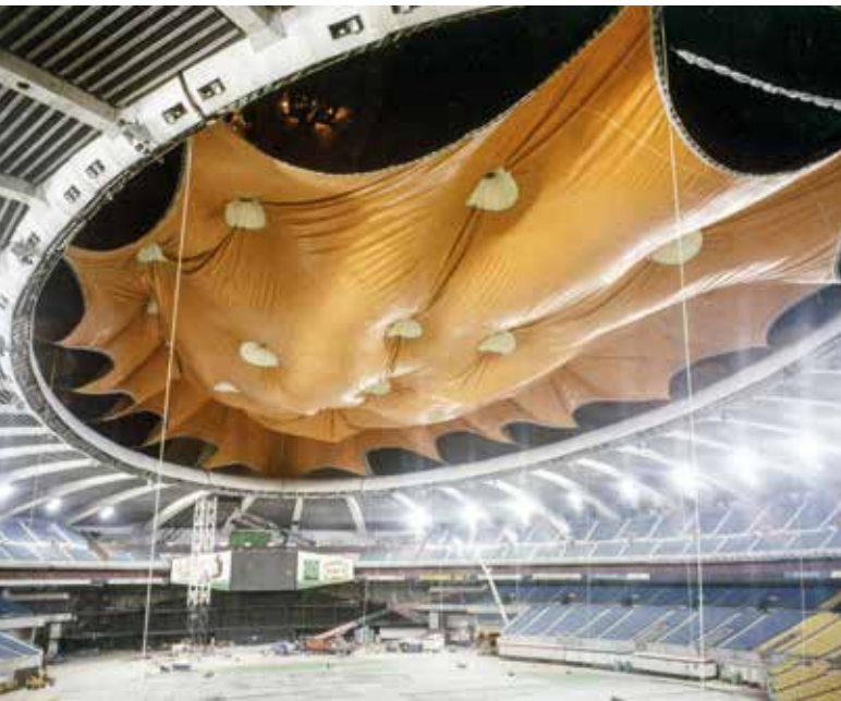
Fig. 5 Raising the Olympic Stadium's retractable roof, April 1987
