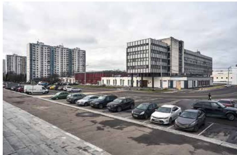
Fig. 9 Moscow Olympic Village, directorate and apartment buildings
