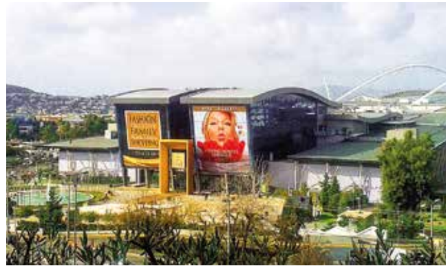
Fig. 2 The IBC transformed into the "Golden Hall" shopping mall, 2012. Source: greece.com
