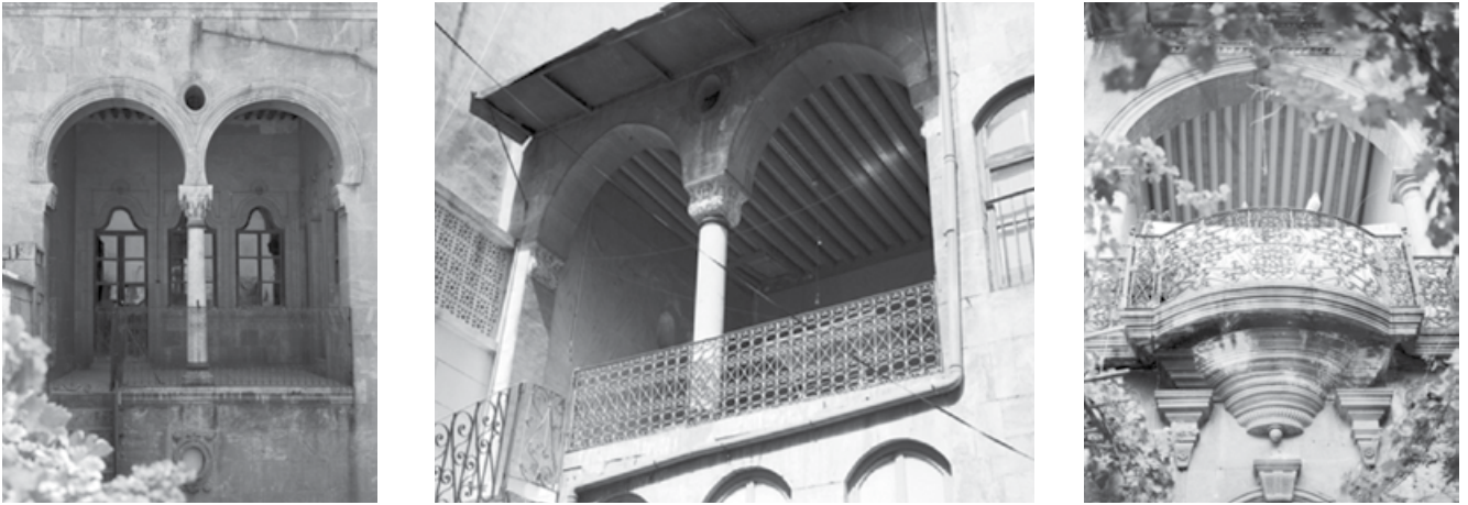
Figs. 11a–c: Selection of photos of traditional courtyard houses in Aleppo (Syrian Heritage Archive, Photos: Jean-Claude David)
