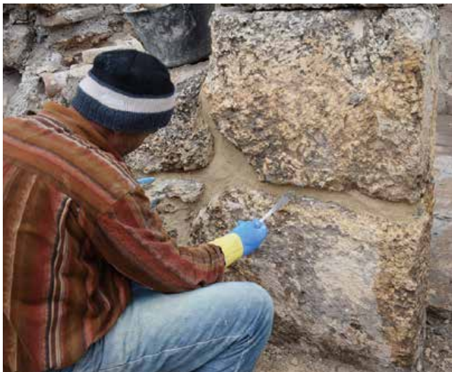
Fig. 10: Baalbek, Bustan Nassif. Joints of rubble stone walls were closed with hydraulic lime coloured with earth (Photo: DAI, Julia Nádor)
