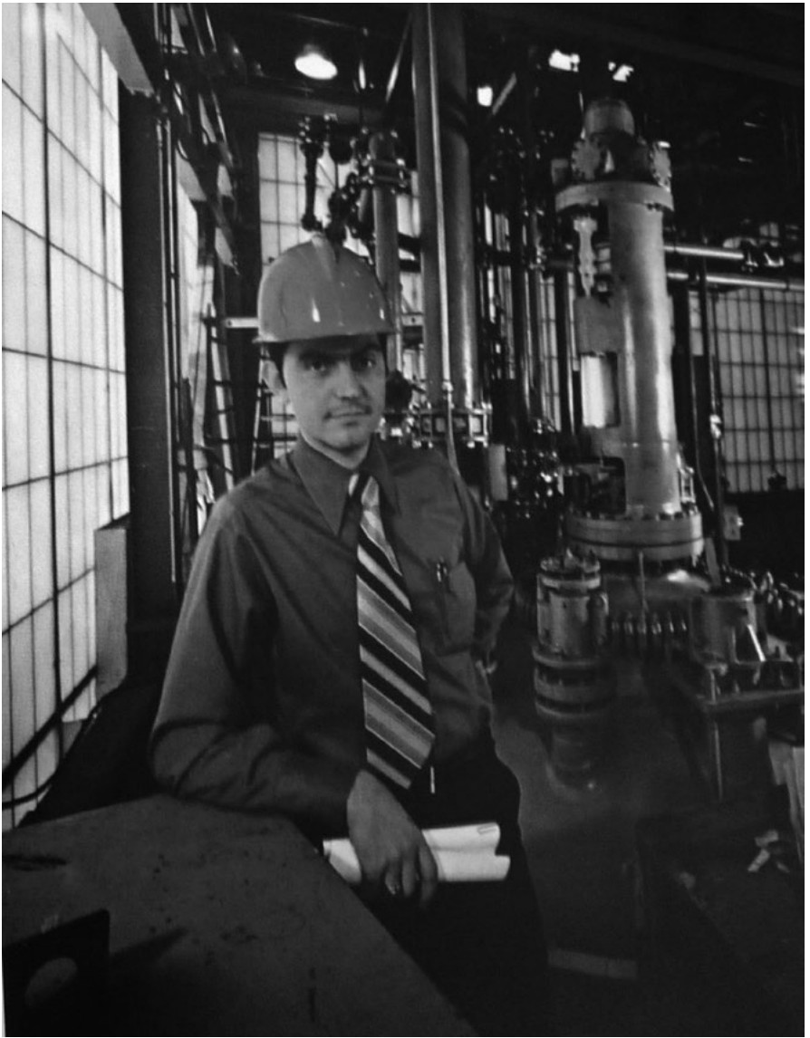
3 John Hill, Robert Marckini, Project Manager of Polaroid's new Chemical Supply plant in Waltham, stands on the facility's third level beside a partially completed reactor system, Fotografie, in: Polaroid Corporation Annual Report for 1970 , hg. v. Polaroid Corporation, Cambridge/Massachusetts 1971
