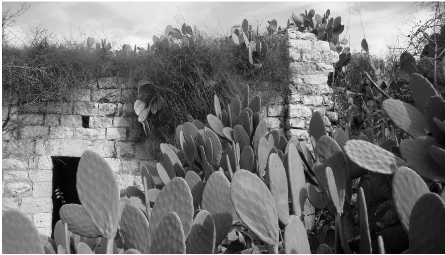
3 Plants struggle through walls of dilapidated houses in Lifta, December 2014.
