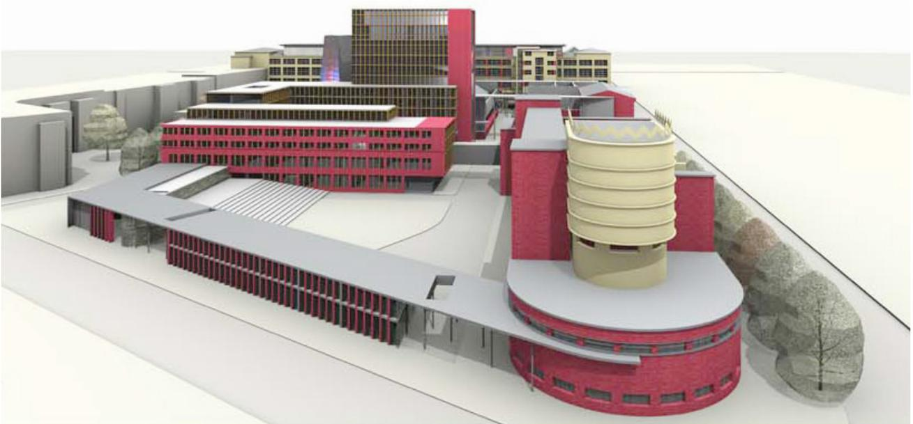
1926–1928; and the dyeing section along Pionerskaya Street, at the beginning of the 1950s), reinforced-concrete frames with central V-shaped ends were used. An end in the form of a ventilation shaft appeared only over one dyeing section, the central one. The reinforced-concrete base of the ventilation shafts in Mendelsohn’s design had been replaced by light metal latticework structures (fig. 3), which were dismantled in the 1970s.
