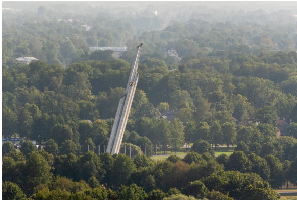
Fig. 7: The demolition of the Victory Monument, 2022. Courtesy of F64 Photo Agency.
