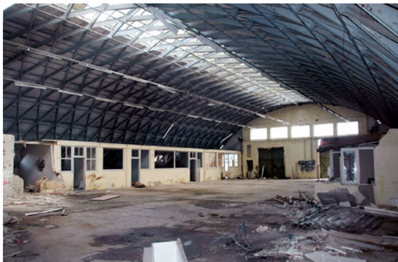
Lamellenhalle in Dessau
