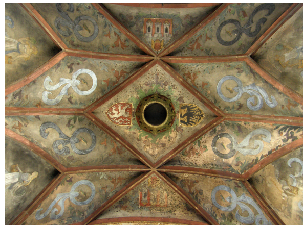
Fig. 6 Old Town Bridge Tower, Vault.
