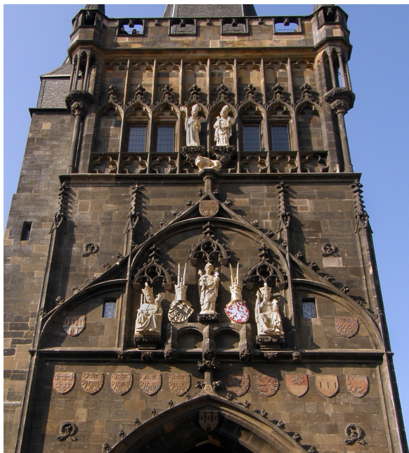
Fig. 5 Old Town Bridge Tower, East Façade.
