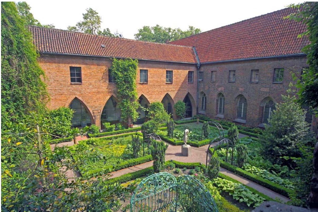
Figure 5: The Museum of Architecture in Wrocław, the cloister garth, 2005
