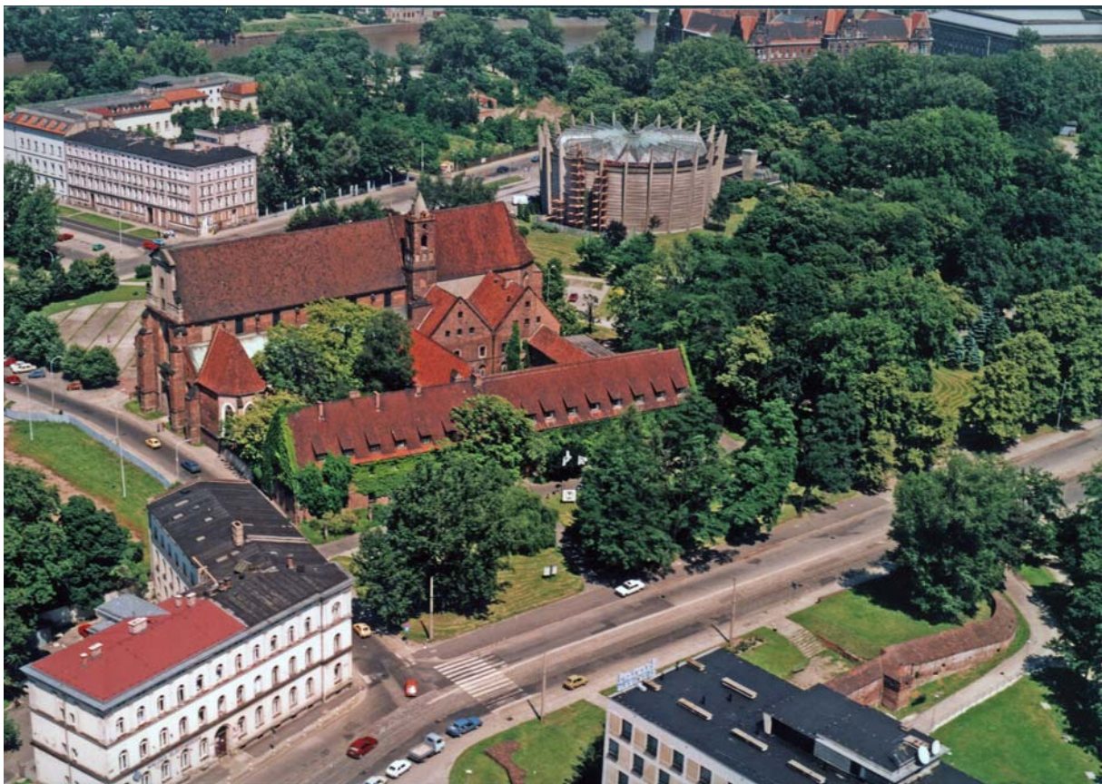
Figure 1: The Museum of Architecture in Wrocław, bird's-eye view, 1997
