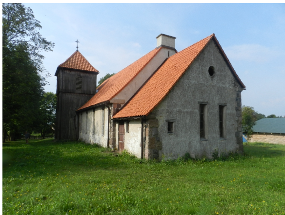
Fig. 7 Evangelic church in Klon by unknown architect (ca. 1935-1937), Photo: 2010
