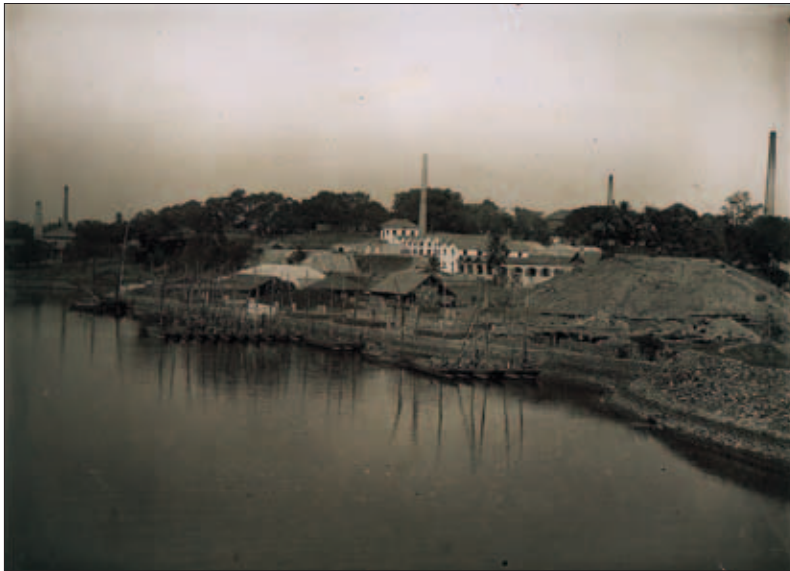
7 Basel Mission Tile Works at Jeppu, Mangalore, Karnataka in a later phase.
