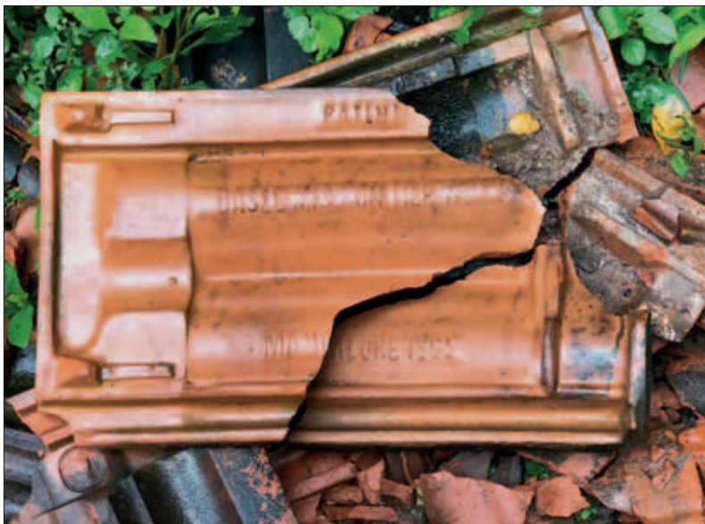
5 Still to be found at Jeppu, Mangalore: used and broken remainder of a standard interlocking tile of the type produced from 1865 onwards in the Basel Mission Tile Works at Mangalore.
