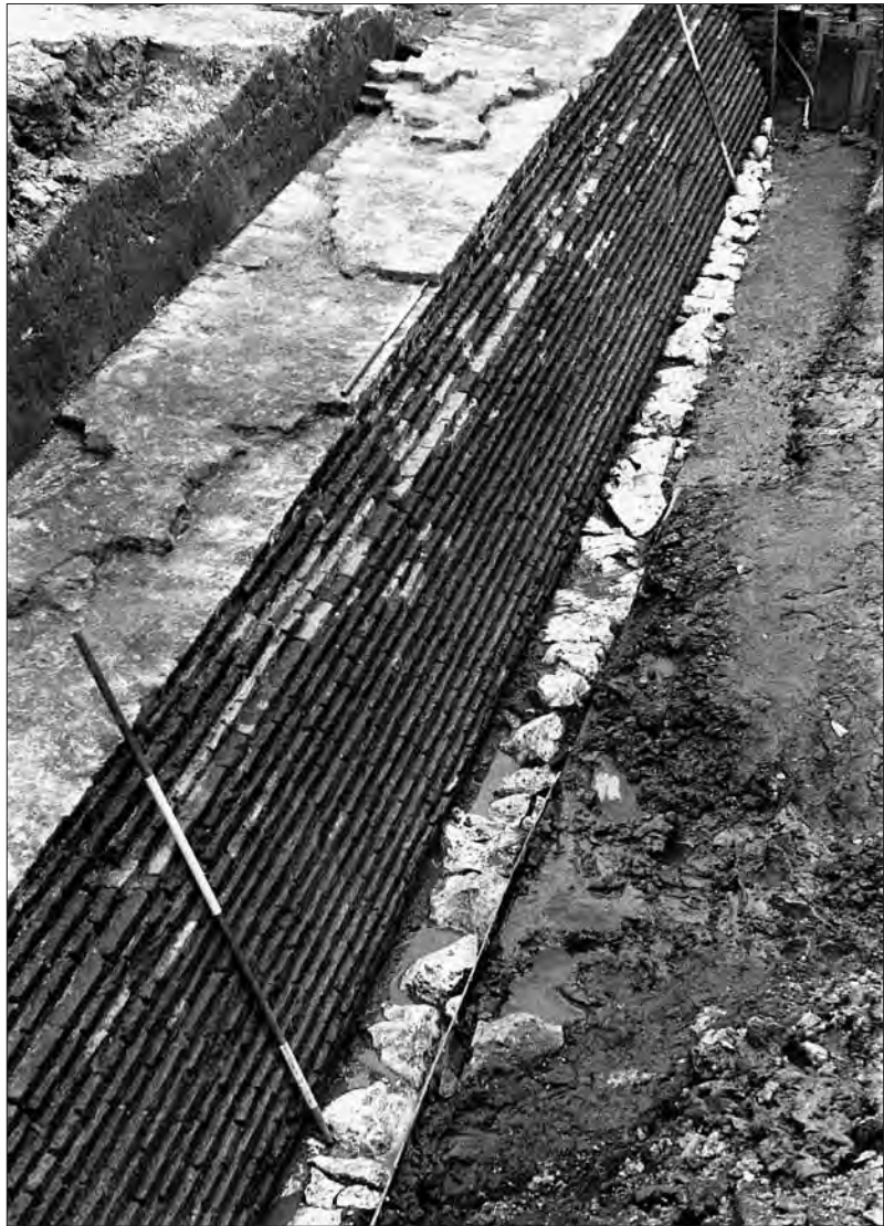
Fig. 2: Part of the medieval Town Wall extending northwards from the Beverley Gate. The lower courses of the Town Wall were battered outwards, and were set on a chalk footing.
