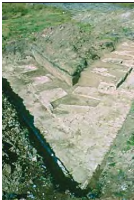
Fig. 5: The Hull Citadel, built between 1681 and 1690. A ravelin at the south-east bastion; the trapezoidal contreforts of the gun positions can be clearly seen lining the walls.
