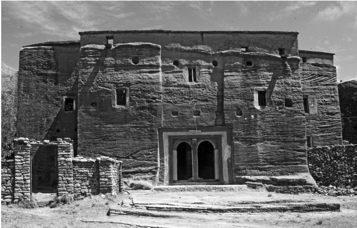
Fig. 7: The rock-hewn 'Tigray cross-in-square' church of Mikael Amba, seen from the west. Its eastern part extends into the solid rock of the mountain..
