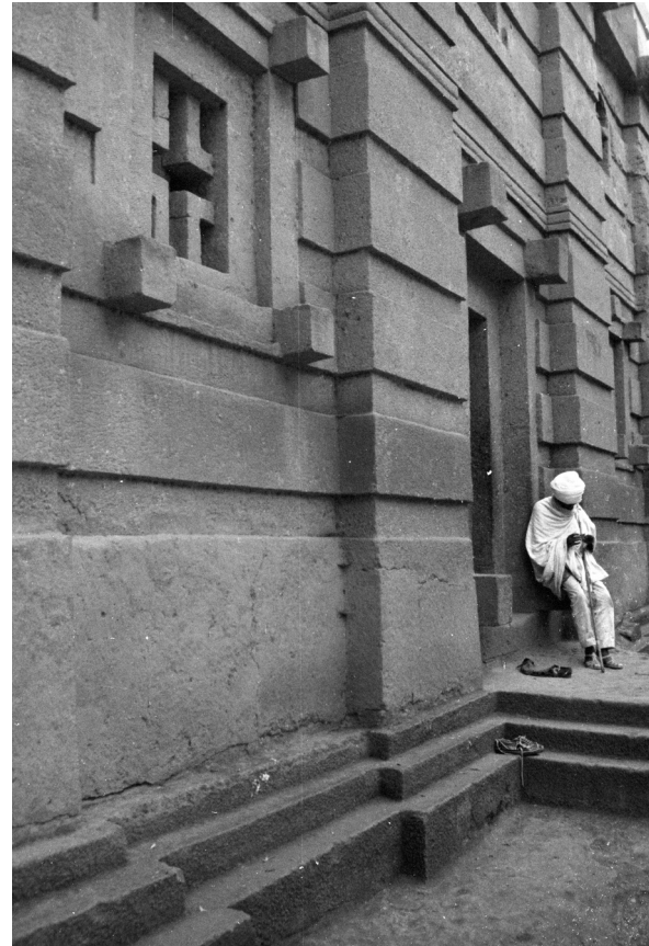
Fig. 9: The ‘monolithic’ basilica Beta Emmanuel at Lalibela. Note the representation of horizontal beams and the form of the doorway, both closely paralleled by the Aksumite stela shown in Fig. 3.
