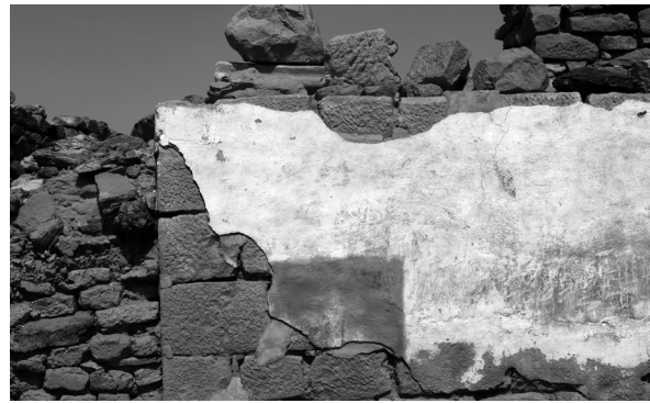
Fig. 9: Southern wall of the North Church during cleaning
