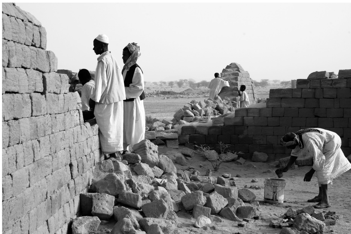
Fig. 22: Covering open wall tops with a lime mortar capping in Complex 500; in the centre and the background walls after treatment (photo: Claudia Näser)
