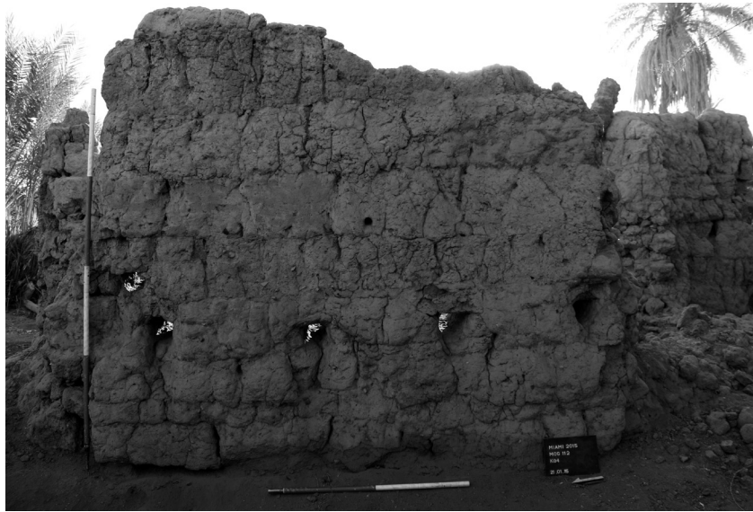
Fig. 30: The western tower at al-Hilla fortress showing beam slots, facing southeast (photo: Rizwan Ahmed)
