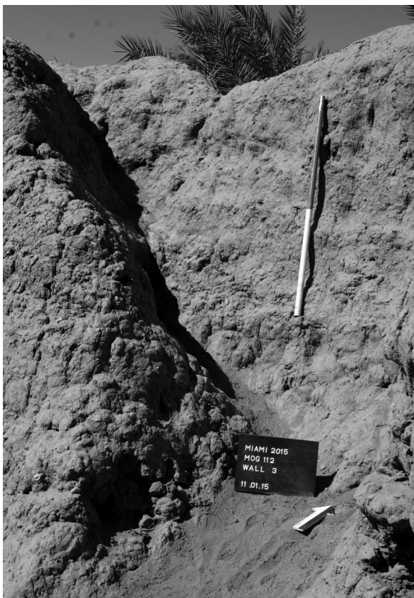
Fig. 29: Remains of staircase at northeastern end of the northwest wall of al-Hilla fortress, facing north (photo: Lisa Seelau)
