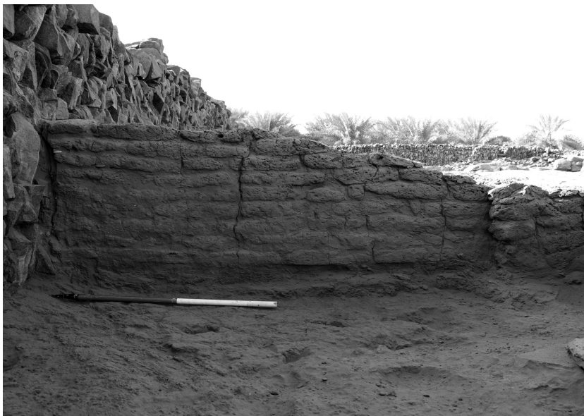
Fig. 10: Mudbrick wall between Spaces 1 and 2, facing south (photo: Gareth Rees)
