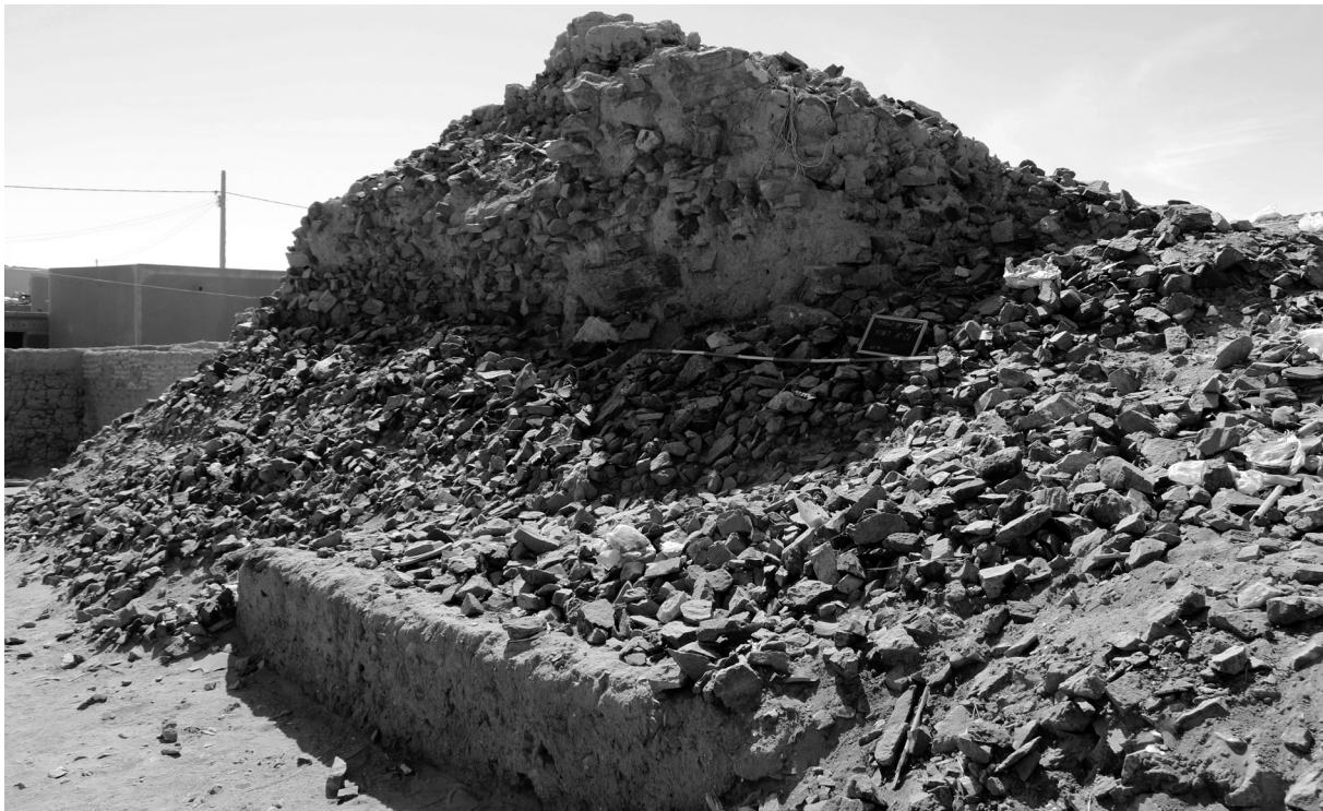
Fig. 11: East wall of fort with modern protection wall added to keep the debris in place (photo Petra Weschenfelder)
