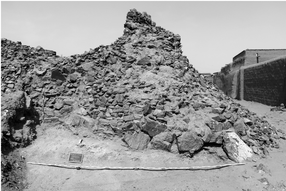
Fig. 5: South view of Southeast bastion (photo Petra Weschenfelder)
