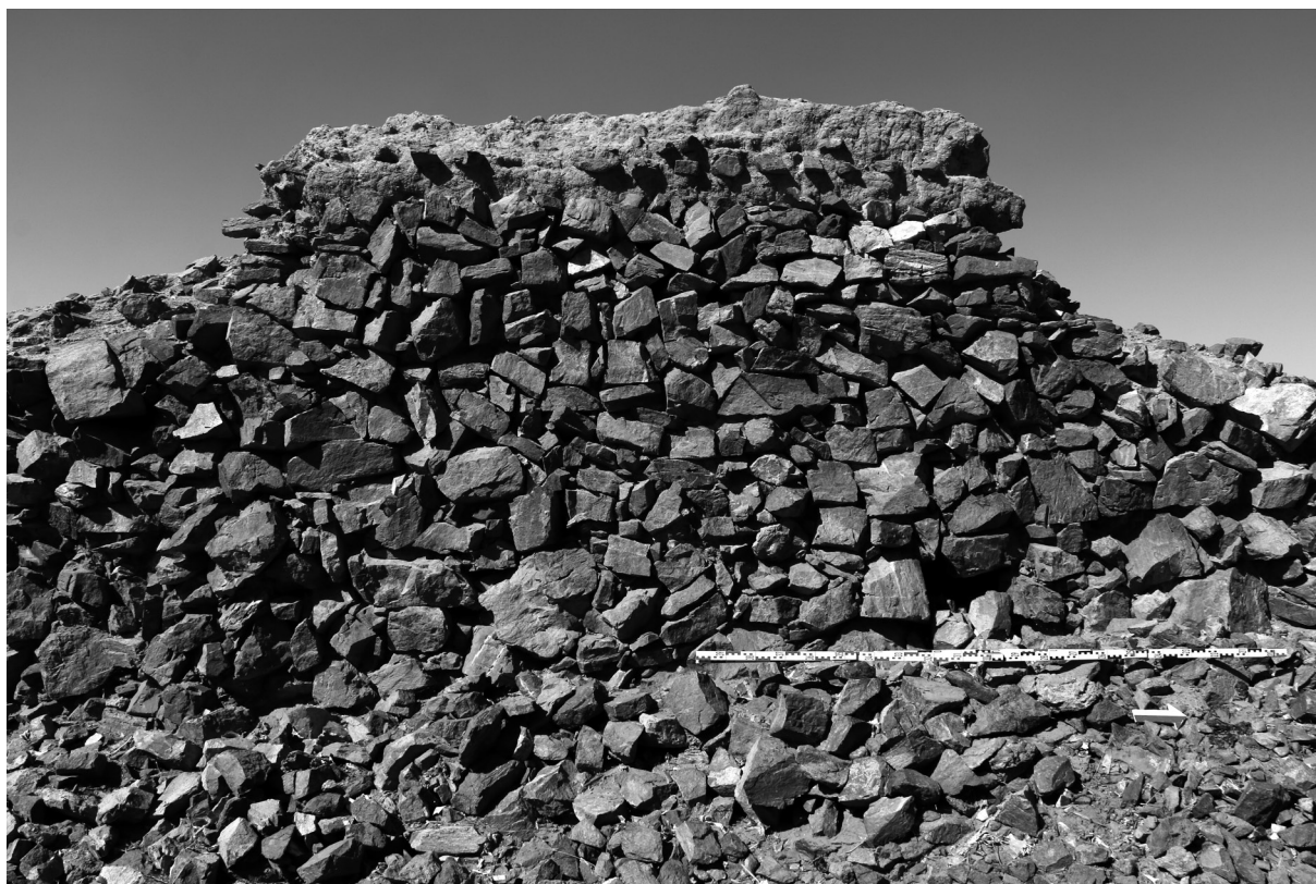
Fig. 4: Exterior of East Wall at southeast end (photo Petra Weschenfelder)
