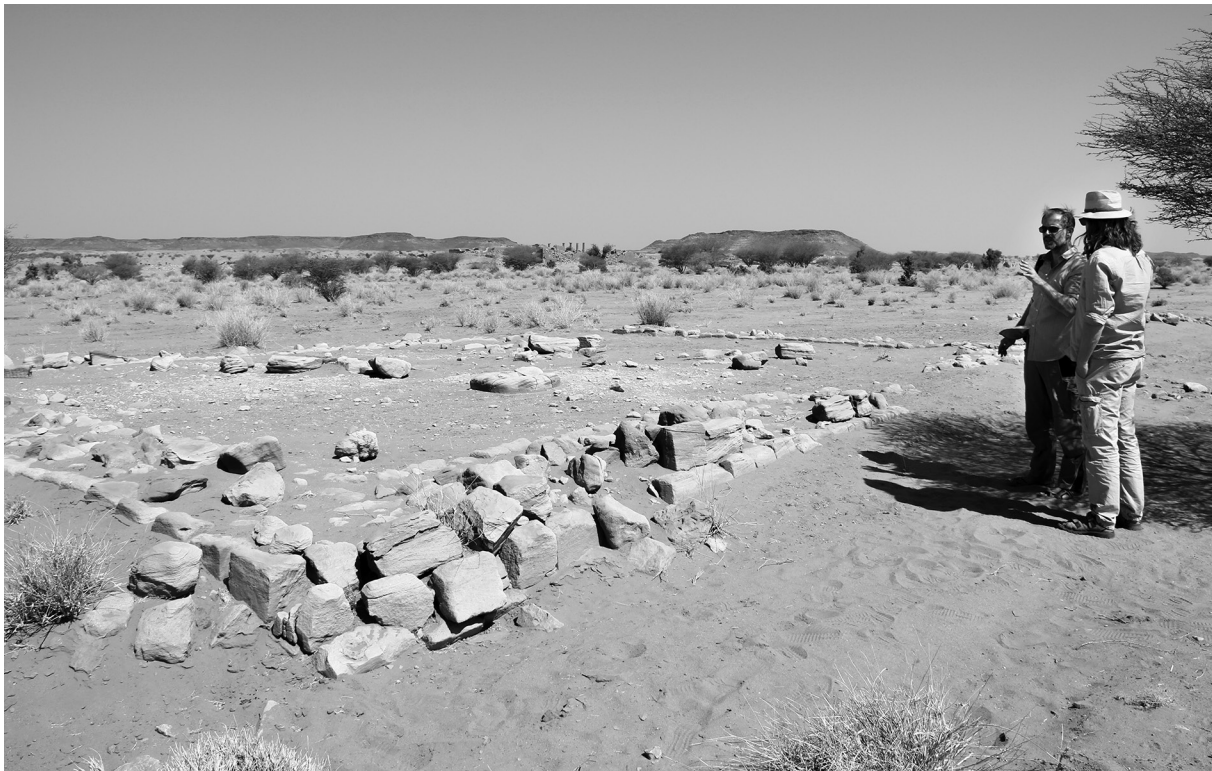
Fig. 2: Conservation survey team during their inspection of Temple ID to the southeast of the Great Enclosure (photo: Cornelia Kleinitz).
