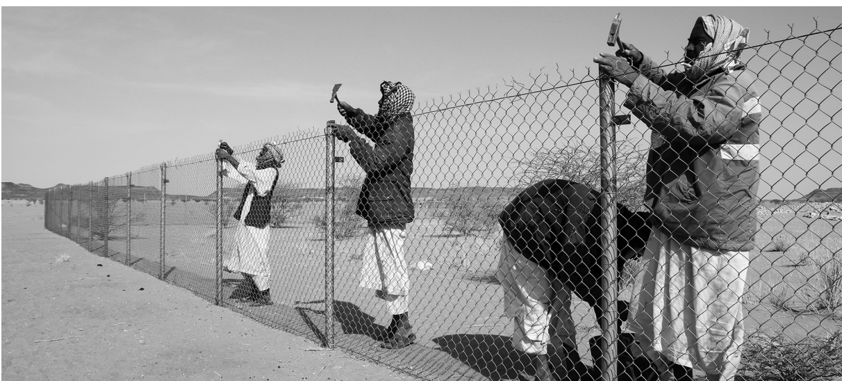
Fig. 33: Closing of the tops of the metal fence poles during the 2017/18 season (photo: Cornelia Kleinitz).
