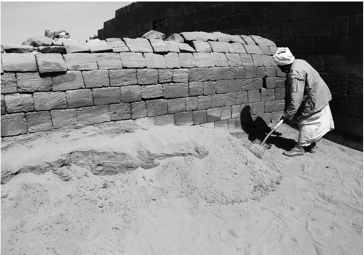
Fig. 36: Removing windblown sand in room 529 of the Great Enclosure (photo: Cornelia Kleinitz).
