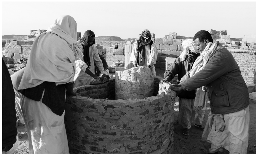
Fig. 19: Demolition of brick enclosure protecting parts of column 5 (photo: Cornelia Kleinitz).
