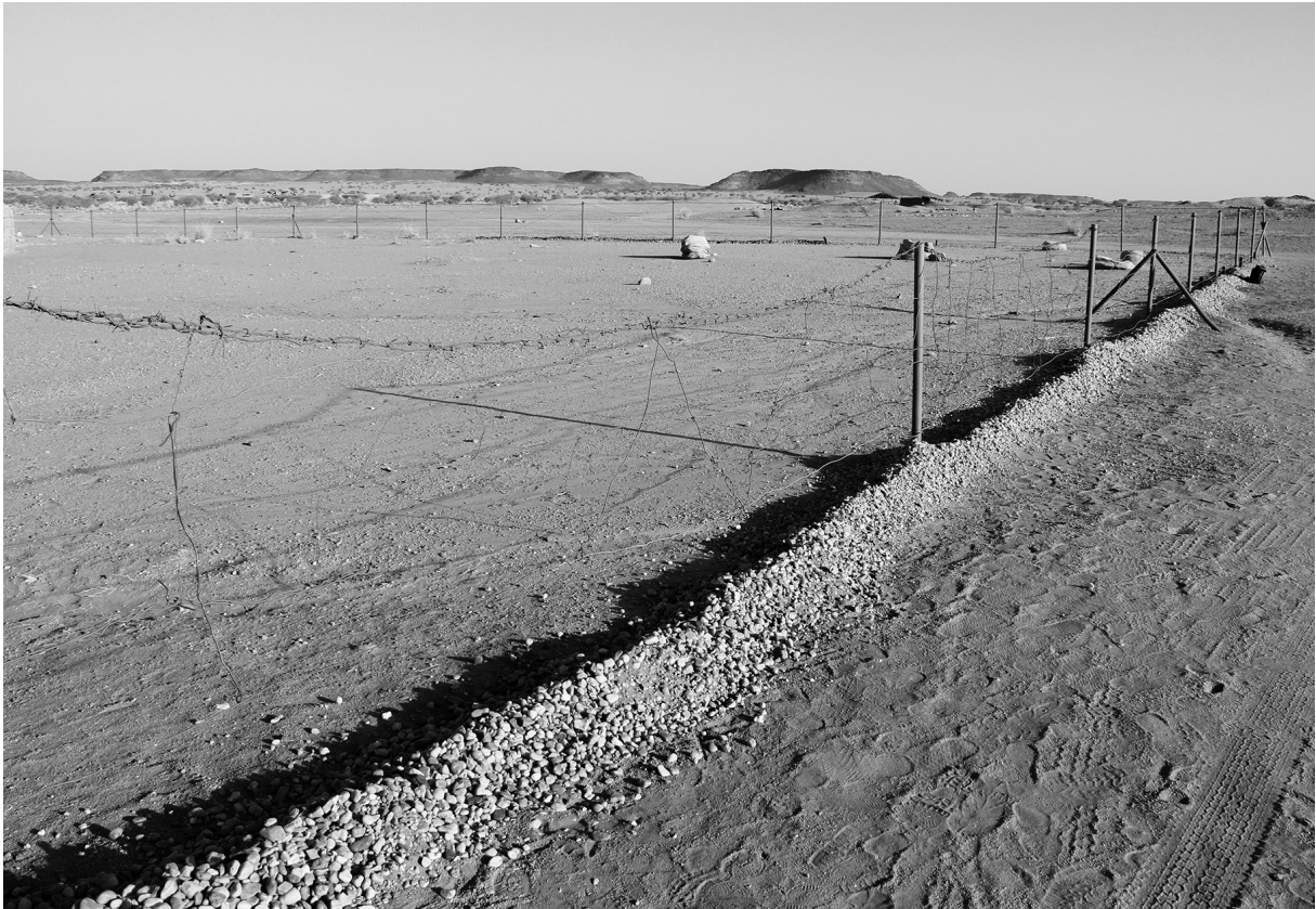
Fig. 35: Fence of the Apedemak Temple after the filling of erosion gullies (photo: Cornelia Kleinitz).
