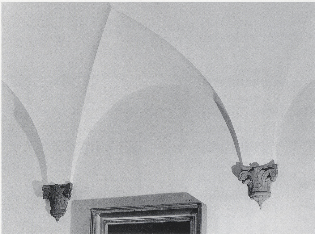
15 Gianfigliuzzi Palace, vaults and corbels in ground floor room [10].
