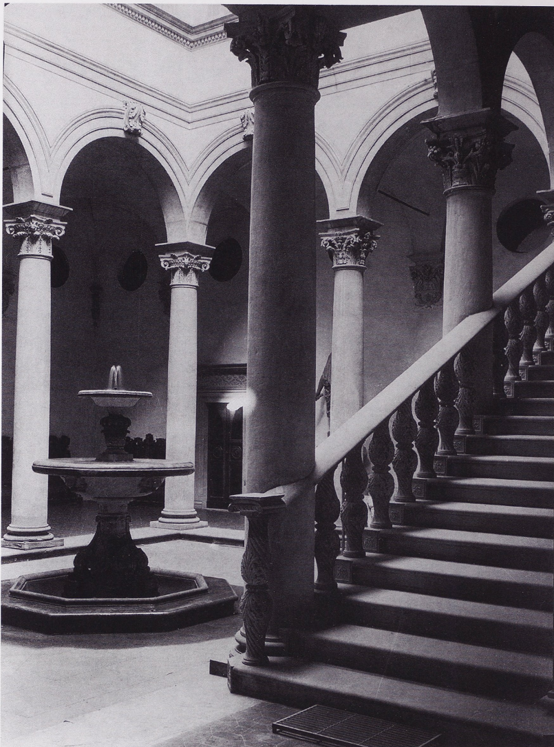
15 Gondi Palace, courtyard.
