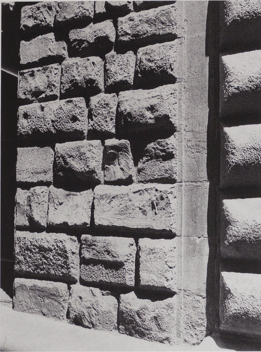
5 Rustication (detail) of Poggi's addition to the Gondi palace along Via Gondi showing the use of the bugnati from the destroyed Giugni palace.
