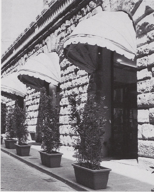
4 Rustication of Poggi's addition to the Gondi palace along Via Gondi showing the use of bugnati from the destroyed Giugni palace.
