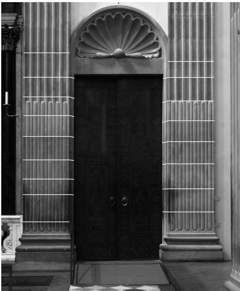
13 Florence, San Lorenzo, southern transept, portal to the Old Sacristy with indication of the joints between the blocks
