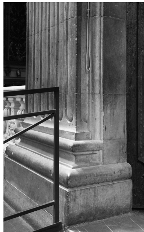
13 Florence, San Lorenzo, southern transept, portal to the Old Sacristy with indication of the joints between the blocks
