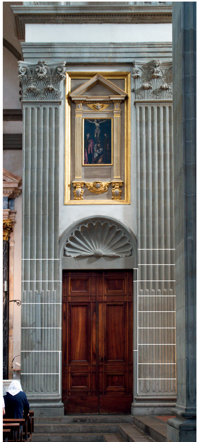
16 Florence, San Lorenzo, northern transept, portal to the Ginori Chapel with indication of the joints between the blocks.
