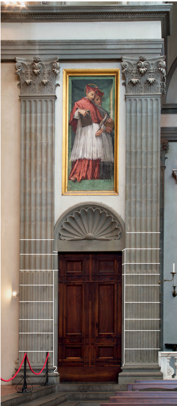
15 Florence, San Lorenzo, southern transept, portal to the Chapel of Cosmas and Damian with indication of the joints between the blocks
