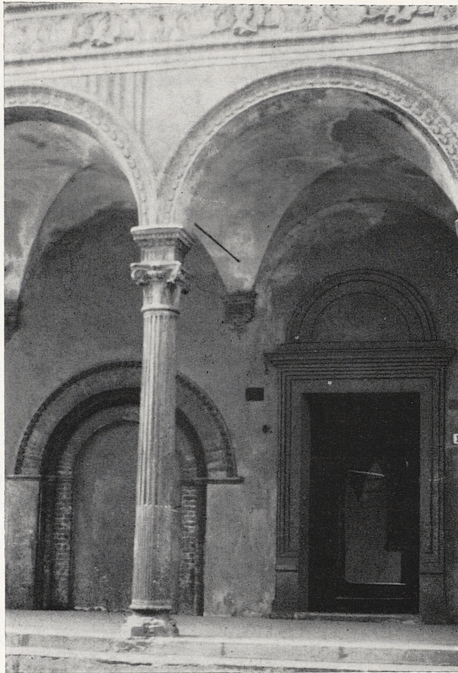
6 View of S. Cecilia showing the portico, the remains of the trecento door and the late 15th century entrance to the vaulted passageway.
