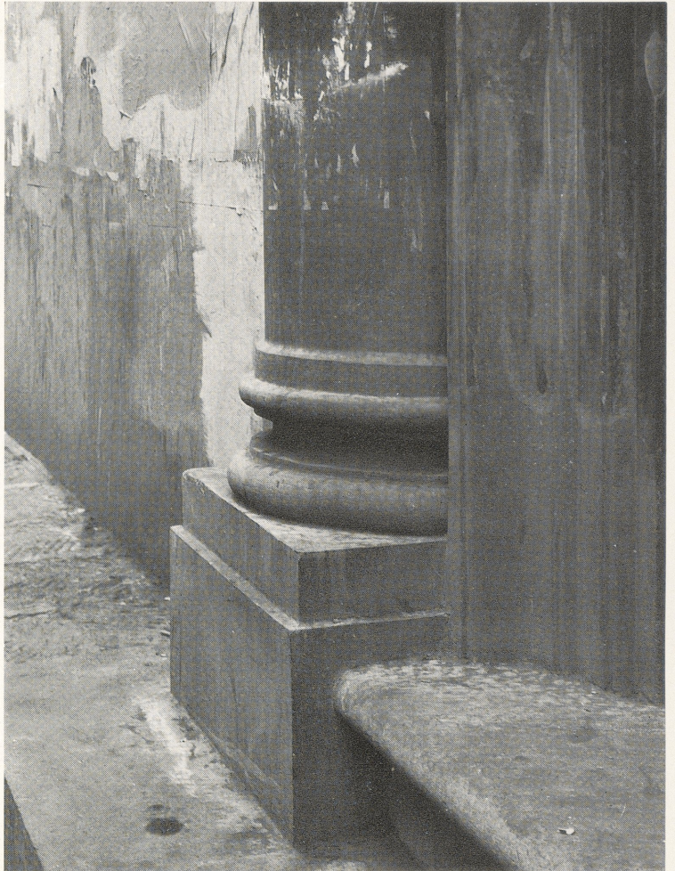
14 S. Apollonia portal, Column basis and steps after 1972 restoration.
