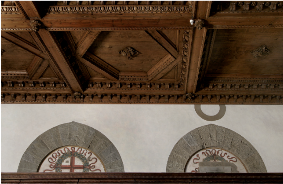
6 Florence, Palazzo Vecchio, Guardaroba, view of circa-1511 windows of the Cancelleria originally overlooking the Cortile della Dogana, walled in during construction of the Guardaroba in 1567.
