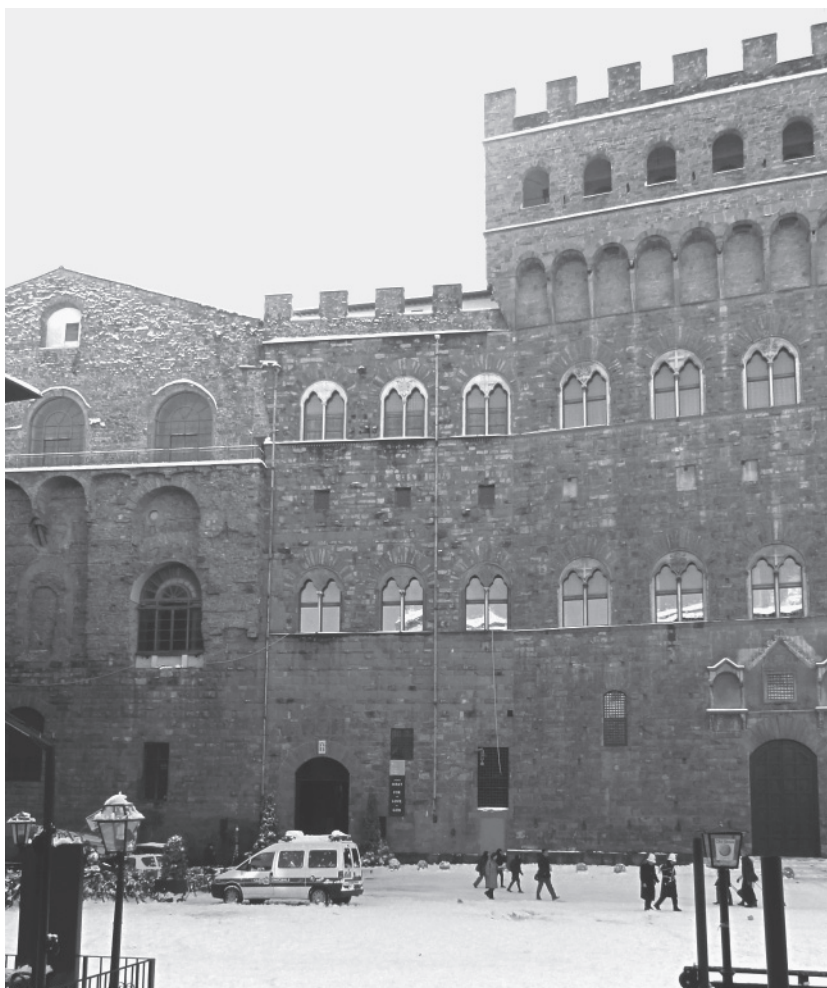
3 Florence, Palazzo Vecchio, northern façade showing c. 1511 construction linking original palace block to council-hall wing.
