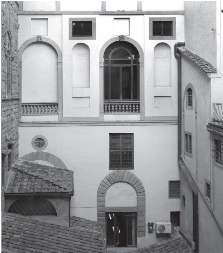
8 Florence, Palazzo Vecchio, Cortile della Dogana, north wall showing walled-in arches following the route of Tasso's destroyed staircase (below) and exterior of Guardaroba (above).
