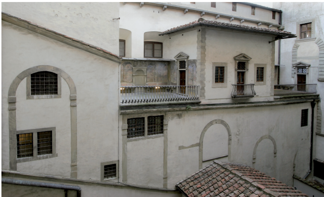
9 Florence, Palazzo Vecchio, Cortile della Dogana, east wall showing walled-in arches tracing the route of Tasso's destroyed staircase.
