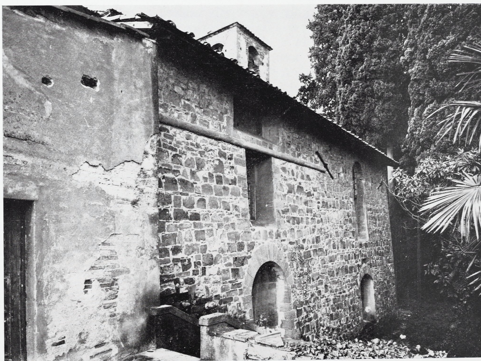
14 The exterior northern wall of Rooms A and B.
