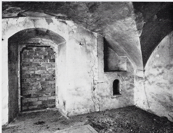
12 The crypt under Room A, partial view (from west).
