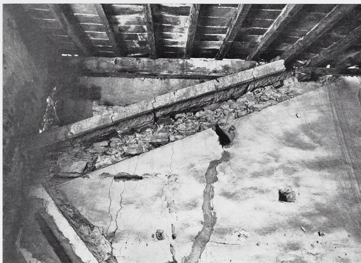
20 The stone gutter on the wall between the Borgherini chapel and the choir chapel of the present church of San Salvatore (see Fig. 2: no. 9).
