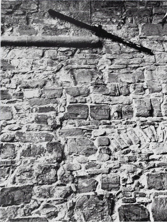
15 Detail of the masonry break on the northern exterior wall of Rooms A and B (see Fig. 2: no. 4).
