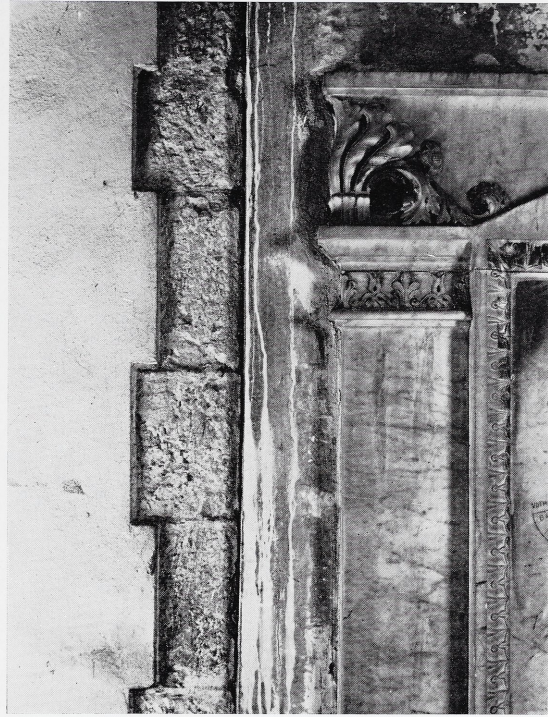
16 Detail of the quoins on the east wall of Room A. These originally defined the exterior northeastern wall of the nave of the 1435 church (see Fig. 2: no. 1).
