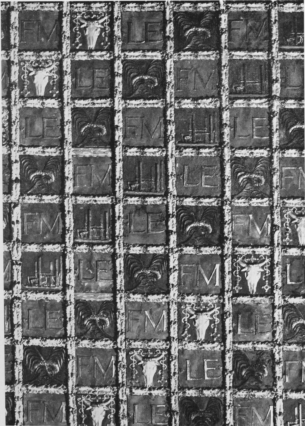
29 Ceiling of the Sala Grande (16th century), piano nobile .
