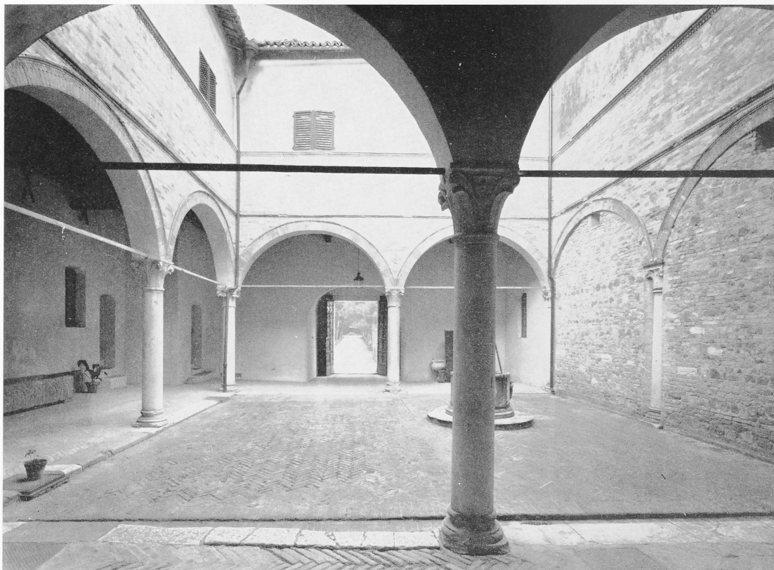
10 Villa Imperiale, courtyard.
