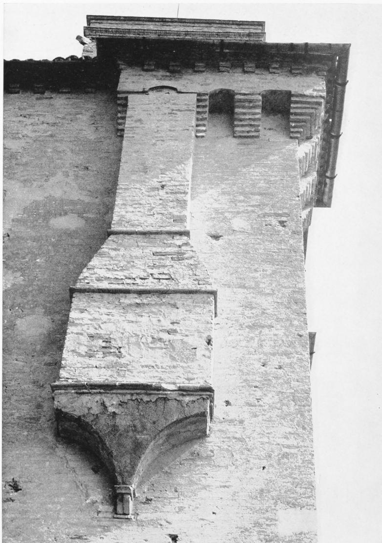
31 Chimney on the south facade.
