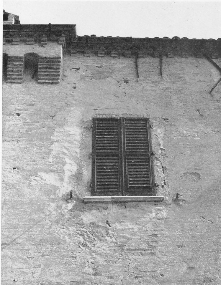
33 Window of the Sala del Giuramento (16th century).
