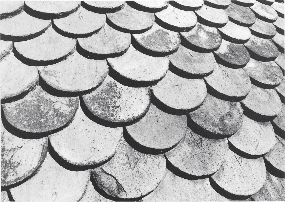
4 Clay Tiles on the Roof of the Medici Chapel.
