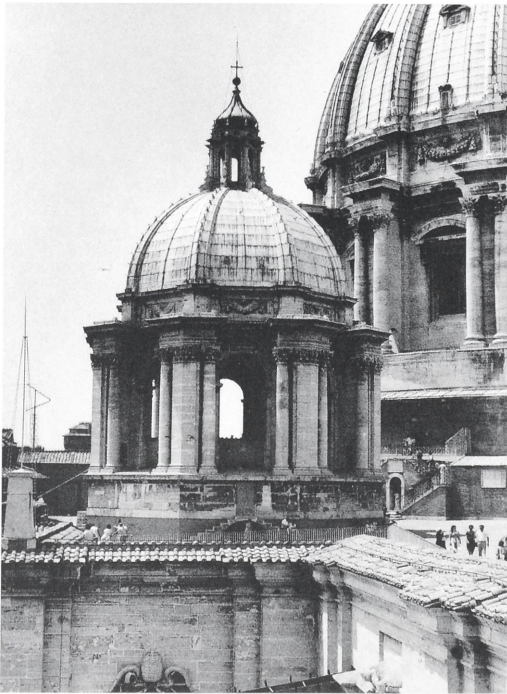
12 Rome, St. Peter's. Lantern and Minor Dome.
