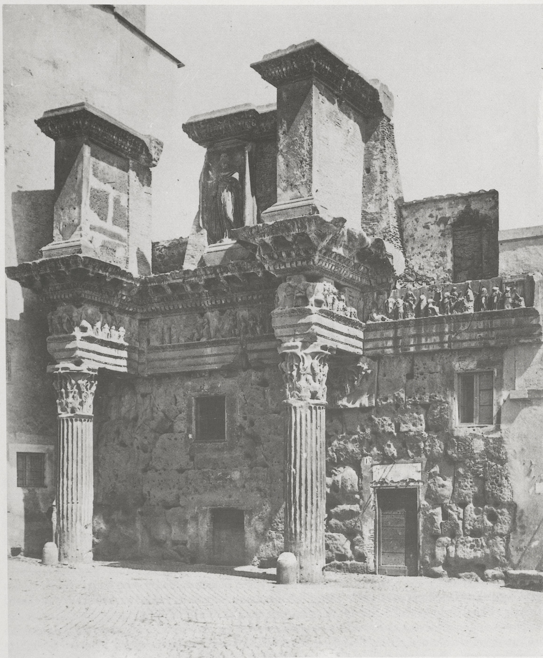
2 Colonnacce, Forum Nervae, Rome. Before the excavation in 1932.
