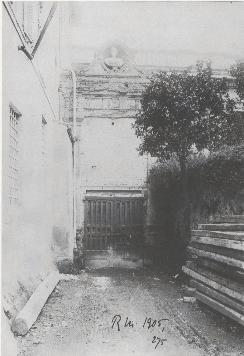
18 Gate formerly leading from Cesi garden to giardino segreto, before 1905.
