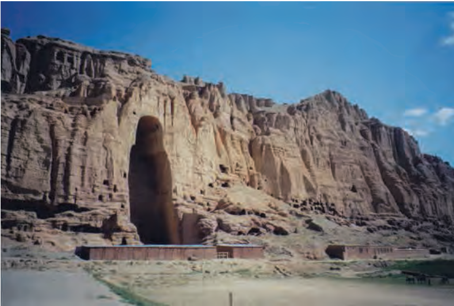
Western Buddha niche with shelters constructed in 2004 and a group of buildings, including the ICOMOS office and a mosque (right), repaired in 2002
