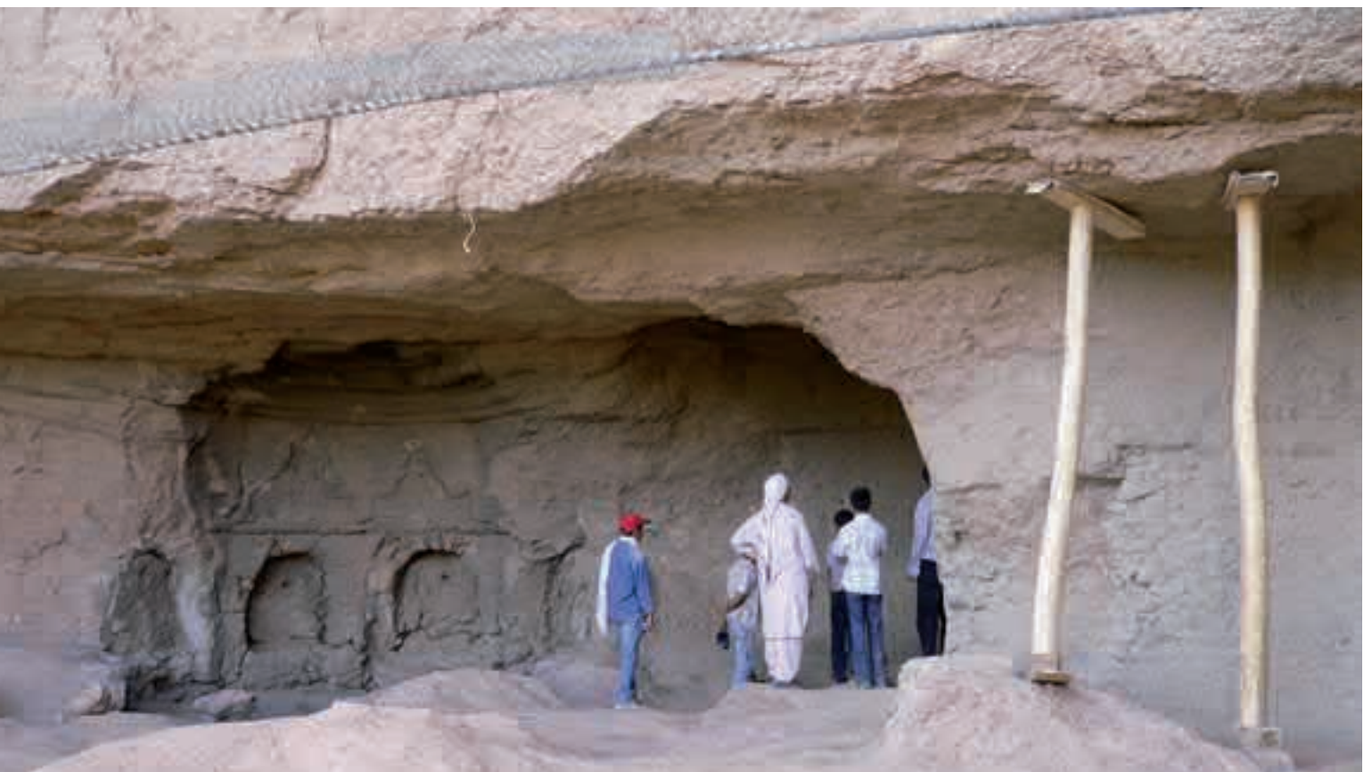
△ Eastern Buddha niche, the ground level with the destroyed caves in the background has been reached ▽ Parts of the niche's back wall had to supported as stone slabs kept on falling down
