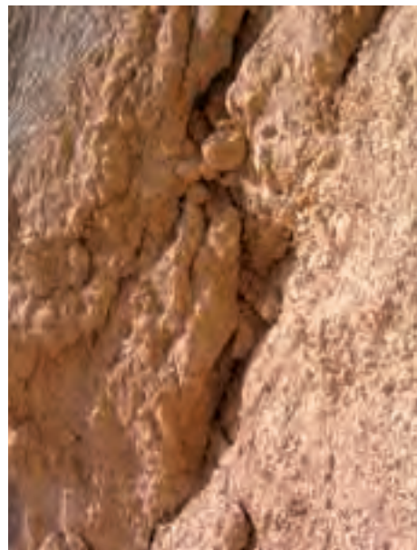
Fig. 22. Left shoulder of the Eastern Buddha (detail of an open joint containing rock debris)
