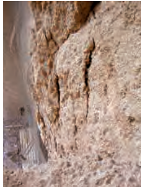
Fig. 21. Left shoulder of the Eastern Buddha (new discontinuities parallel to the back wall)
