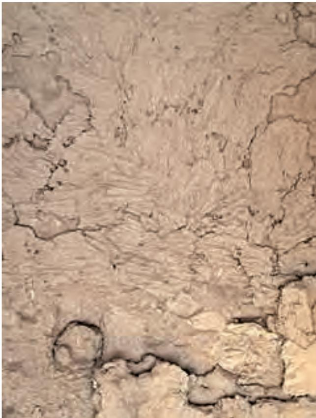
◁ Eastern Buddha, preserved original clay plaster areas (marked in yellow); in total about 21 square metres, secured in 2008 by gluing and needling
