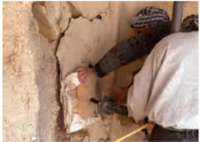
Original clay plaster fragments (right side of the Eastern Buddha), preparation for the setting of anchors: Mujtabah Mirzai drilling a hole into an existing bullet hole for an anchor. ▷▷▷
