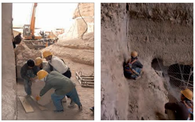
Removal of rock fragments with a heavy-duty crane (left). The steps near the Buddha's shoulder are cleared of rubble so that a temporary base for the upper zone of the scaffold can be added (right).
