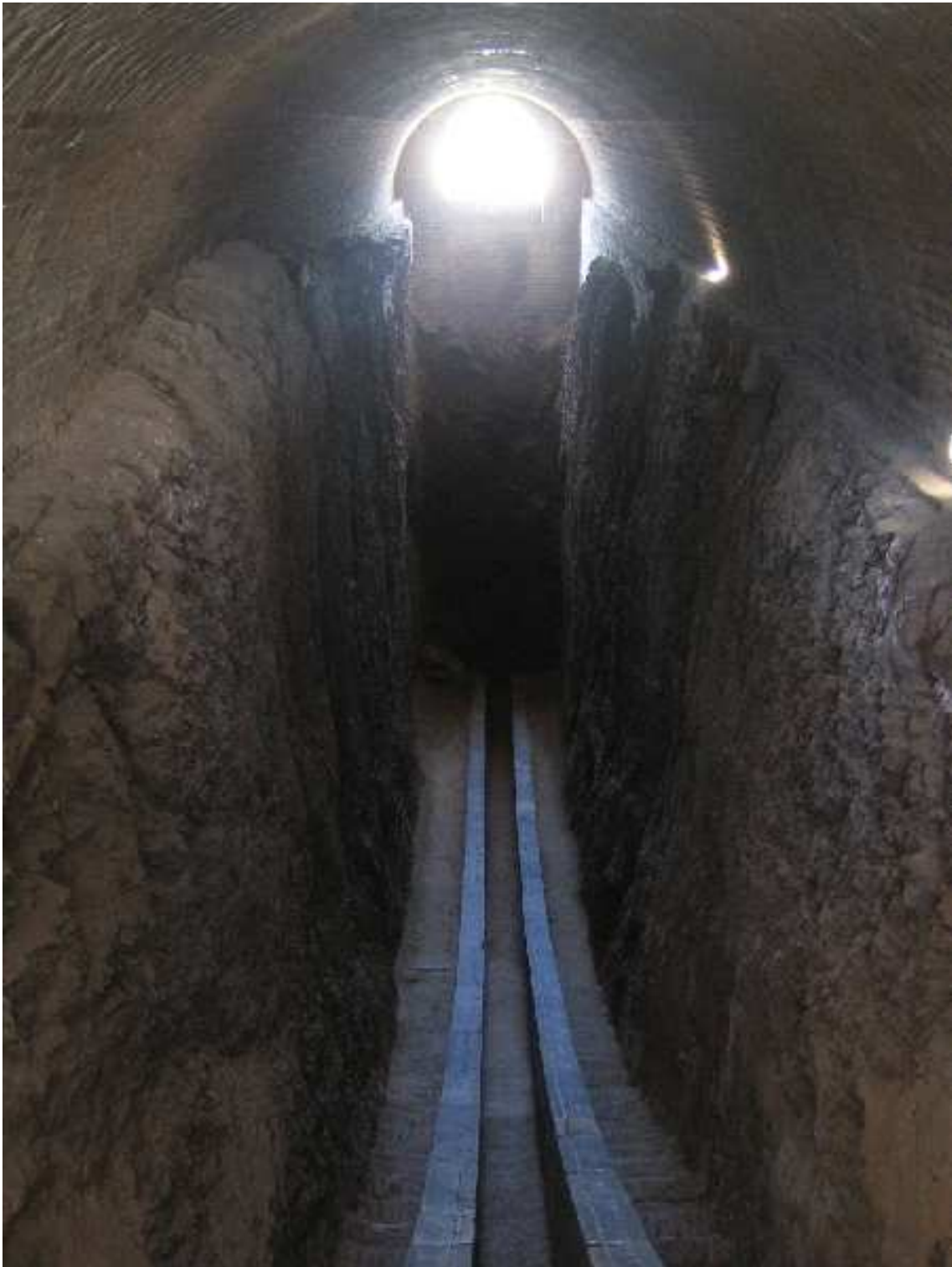
Figure 3.1: Uluğ Begs (1394–1449) sextant of 40 m radius, Samarkand Observatory, Uzbekistan (©UNESCO)
