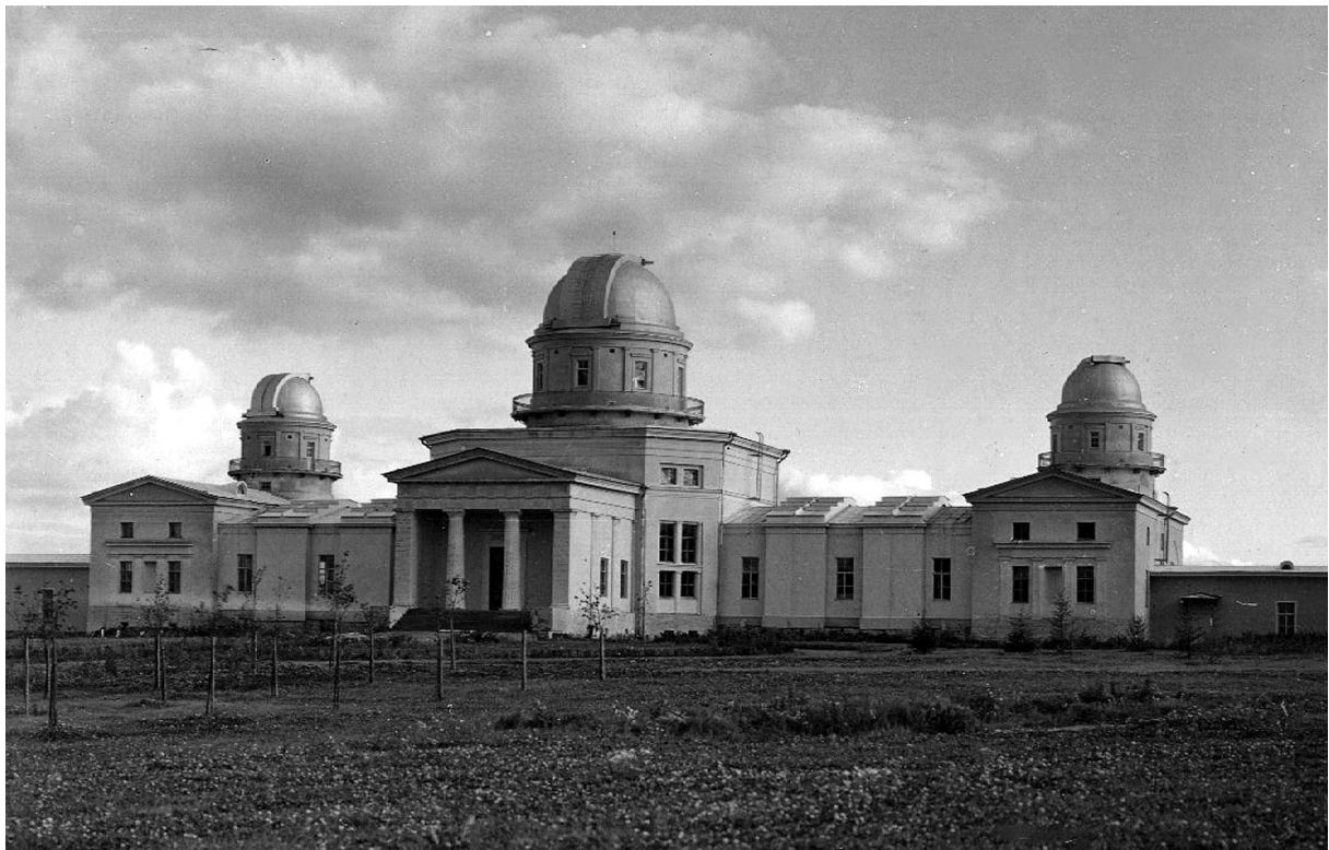
Figure 6.1: Above: The Nicholas Central Astronomical Observatory (Pulkovo Observatory) (the view before WWII) Below: The restored Pulkovo Observatory (the view after WWII) (Pulkovo Observatory, St. Petersburg)
