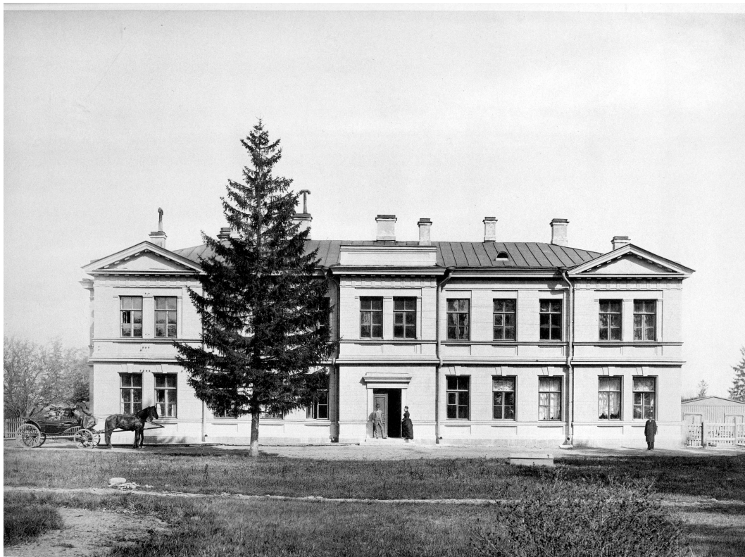
Figure 6.10: Above: The Plan of the Ground Floor of the Astrophysical Laboratory Below: The Astrophysical Laboratory, architect Alexander F. Vidov (1886) (Pulkovo Observatory, St. Petersburg)
