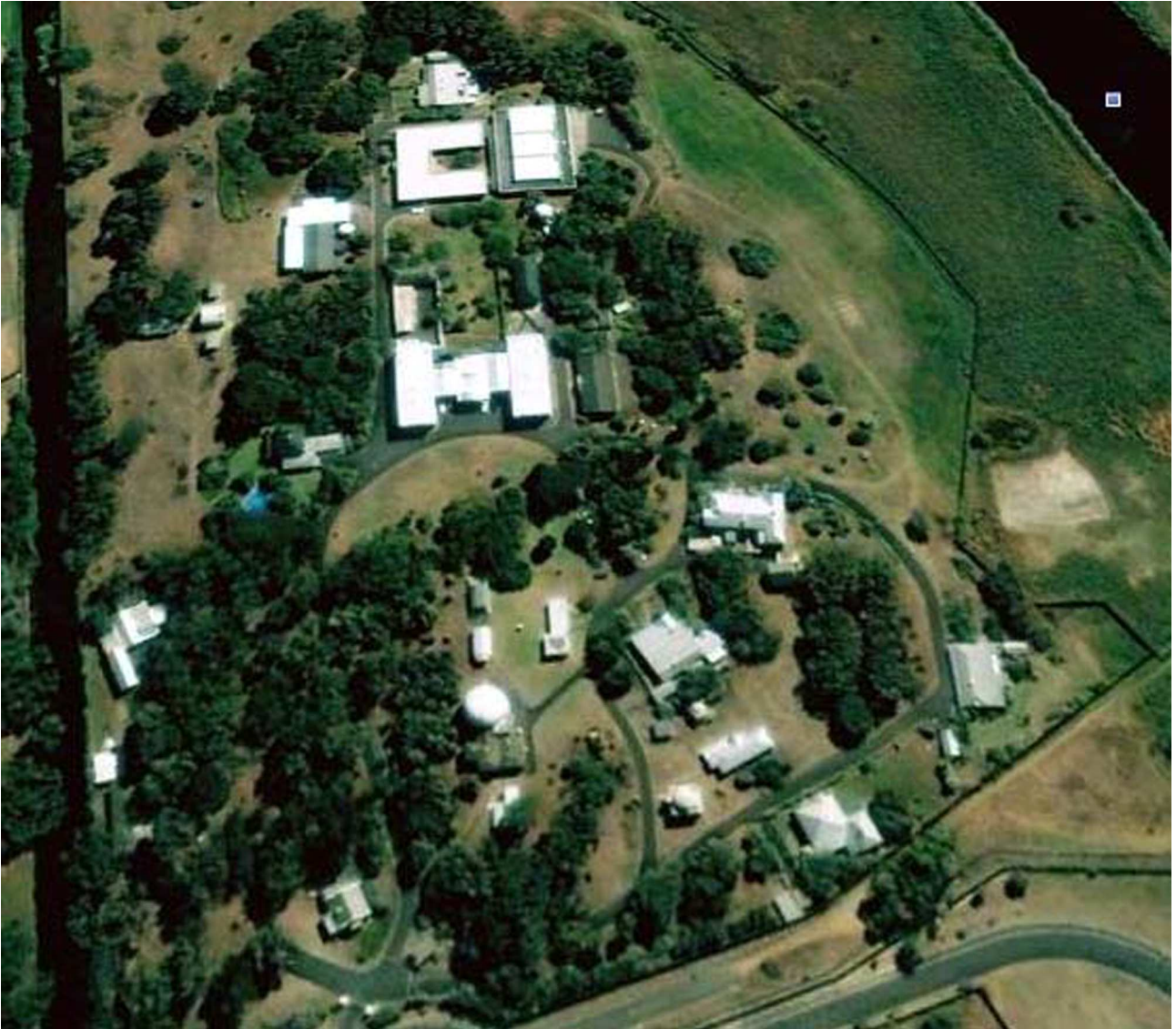
Figure 22.1: Google image of Royal Observatory, Cape of Good Hope. The H-shaped main building was completed in 1828
