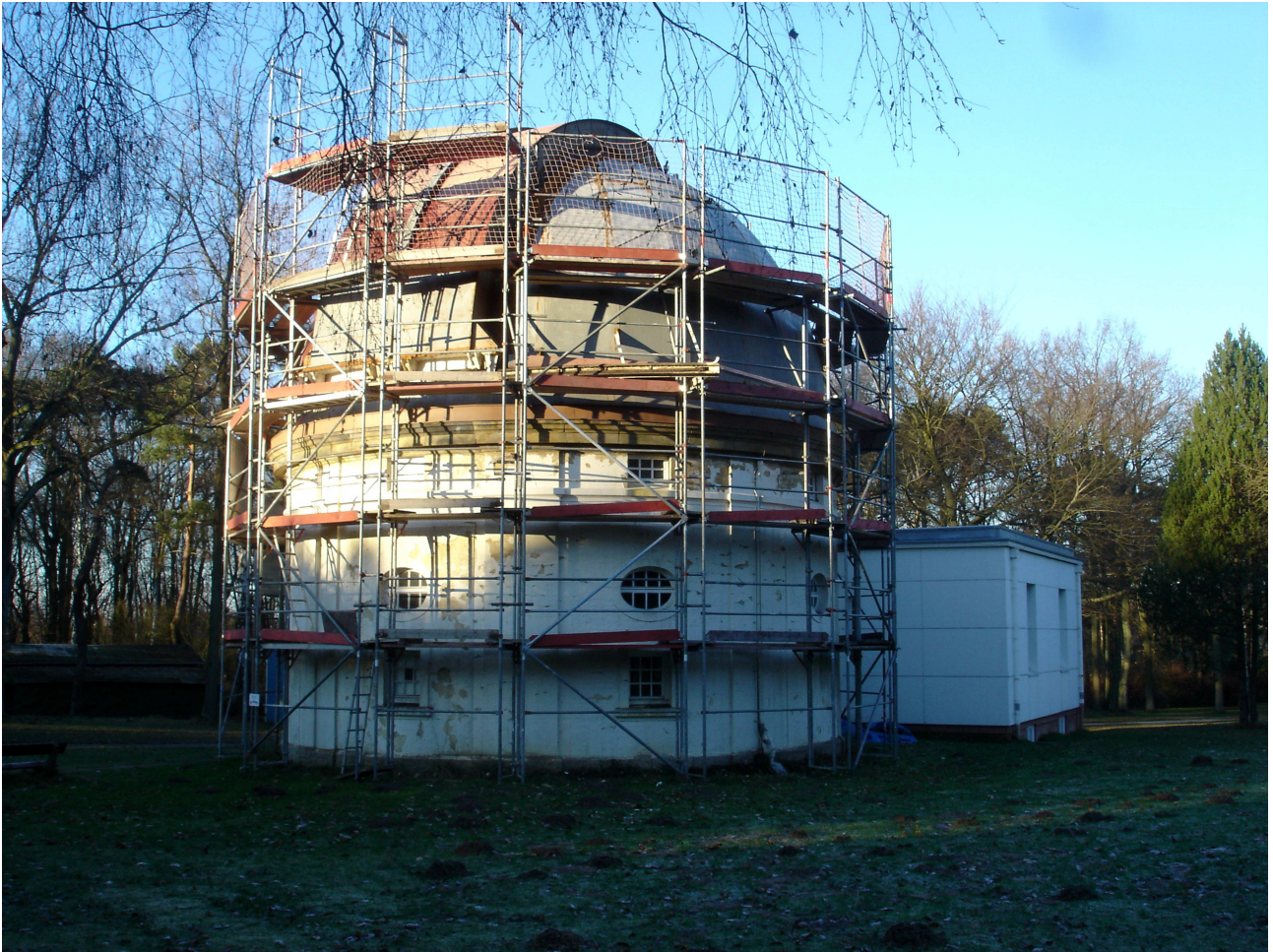
Figure 39.1: Restoration of the 1m-reflector building (Photo: Gudrun Wolfschmidt)
