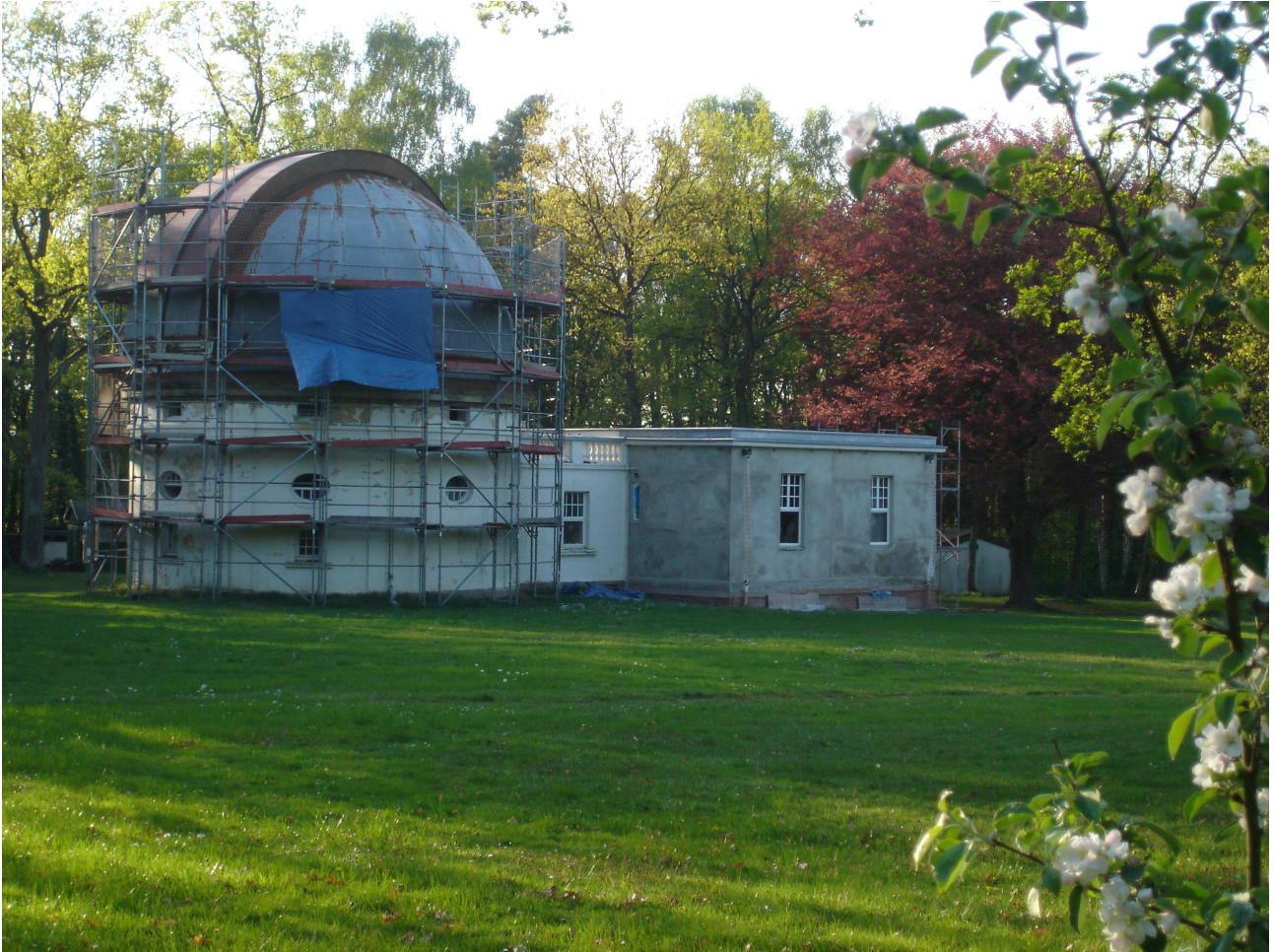
Figure 39.4: Restoration of the 1m reflector building (2008–2009) (Photo: Gudrun Wolfschmidt)
