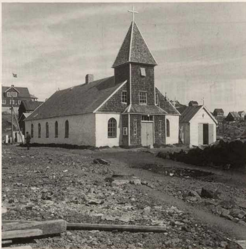
The principal work of the stone building area in Greenland is undoubtedly the big church in Maniitsoq (formerly Sukkertoppen). The church has been converted into a library.
