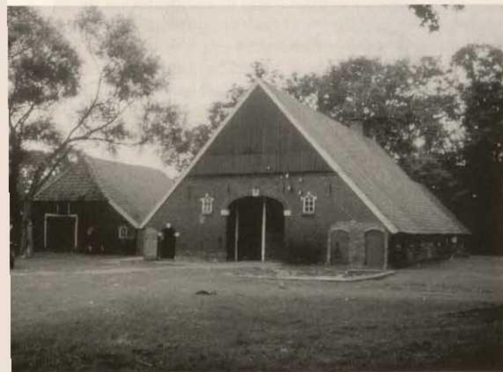
Hall farm building tradition: farm at Eibergen, Gelderland. The building to the right contains both dwelling area and working part. The second building is a separate barn. Photo: SHBO.
