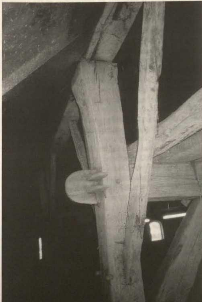
Detail of anchor beam framework of hall farm group. Photo: SHBO.
