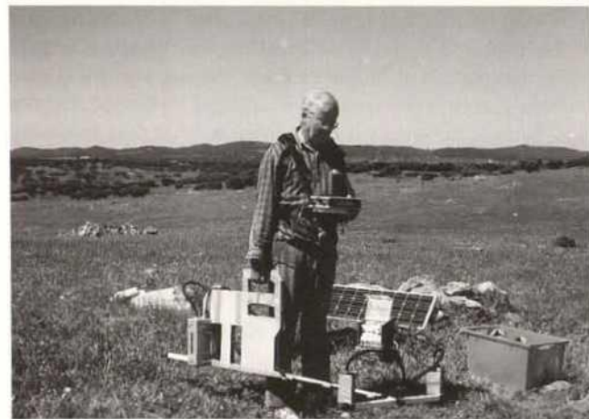
Fig. 2 and 3. Monte da Ponte 1994. Caesium magnetometer Picotesla-system CS2/MEP720 (Scintrex/Picodas) at first application in March 1994
