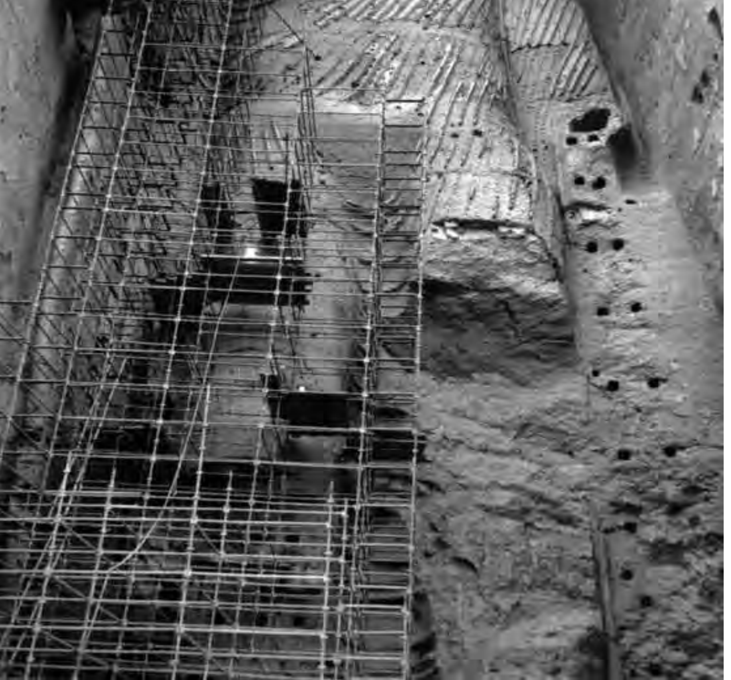
Fig. 26. The Western Buddha during restoration (photo: ASI)
