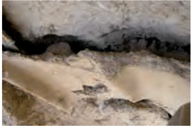
△ Clay plaster fragments in situ at the Eastern Buddha: loosened after the explosions, partly detached from the rock surface and in danger of falling off
