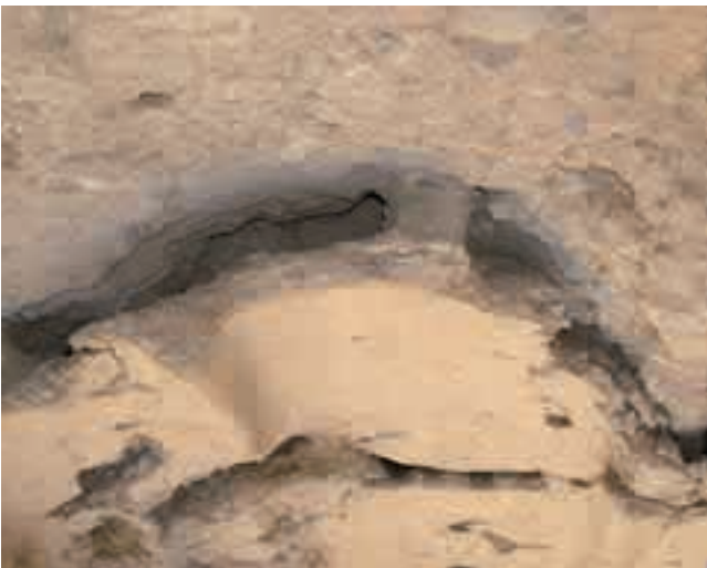
▽ ▽ Clay plaster fragments in situ at the Eastern Buddha, spot-bonding with clay-gypsum mixture
