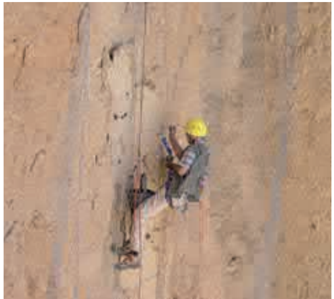
△ Clay plaster fragments in situ at the Eastern Buddha: loosened after the explosions, partly detached from the rock surface and in danger of falling off
