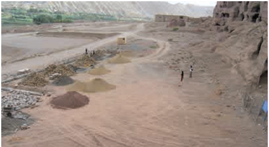
The construction of the shelters begins.
