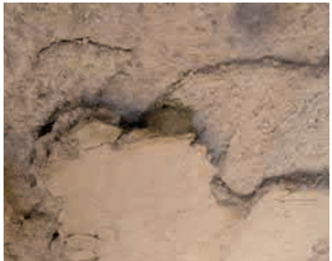
▽ ▽ Clay plaster fragments in situ at the Eastern Buddha, spot-bonding with clay-gypsum mixture
