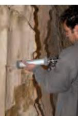
Bonding of clay plaster fragments; by means of a splaying apparatus pressure is carefully put on the clay plaster fragments; on the left underneath the arm hole.  $\triangleright \triangleright$
