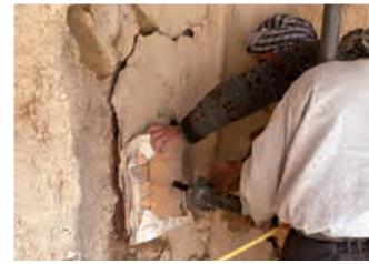
Original clay plaster fragments (right side of the Eastern Buddha), preparation for the setting of anchors: Mujtabah Mirzai drilling a hole into an existing bullet hole for an anchor.  $\triangleright\triangleright$
