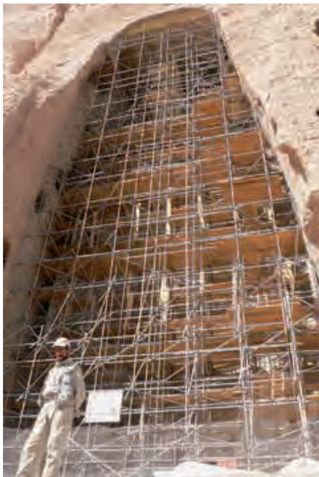
The completely scaffolded Eastern Buddha niche
