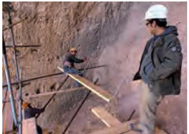
Bracket-like cantilevers are added to the scaffold so that the niche's back wall can be reached
